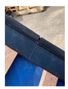
4, Once all the slate verge is installed start laying the slates ensuring that they are fixed into the overlap of the verge unit.
