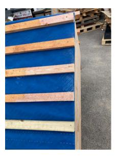
2, Install the Cromar Dry Fix Slate Verge directly on top of the battens allowing for a 50mm overhang at the eaves into the gutter and so not to obstruct the gutter the end of the Slate verge may need trimming underneath.
